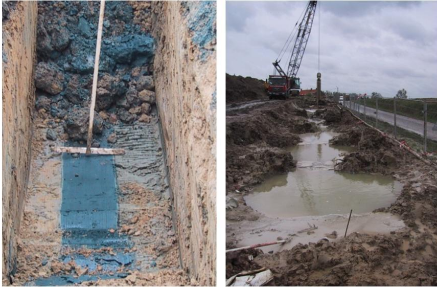
Figure 6 : Construction of the circular impermeable cement-bentonite slurry wall
