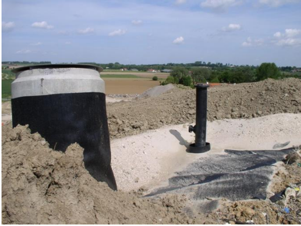
Figure 18 : Construction of landfill gas extraction well
